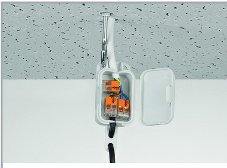
Pendant light connection in a suspended ceiling
